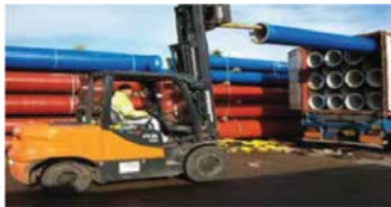
Loading with forklifts using boom attachment
