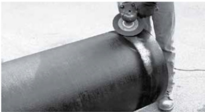
Surface coating removed at the place of welding
